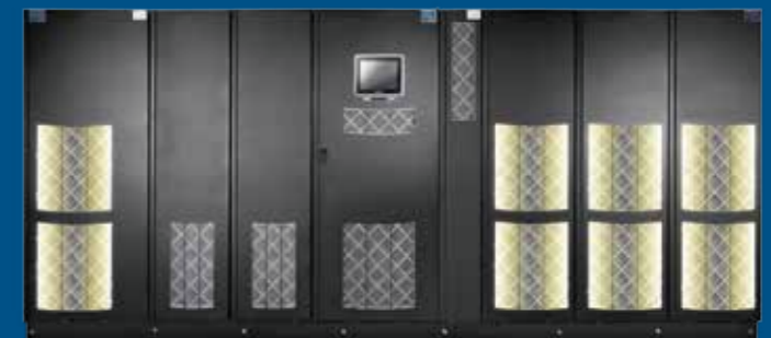
9395P on batteries
