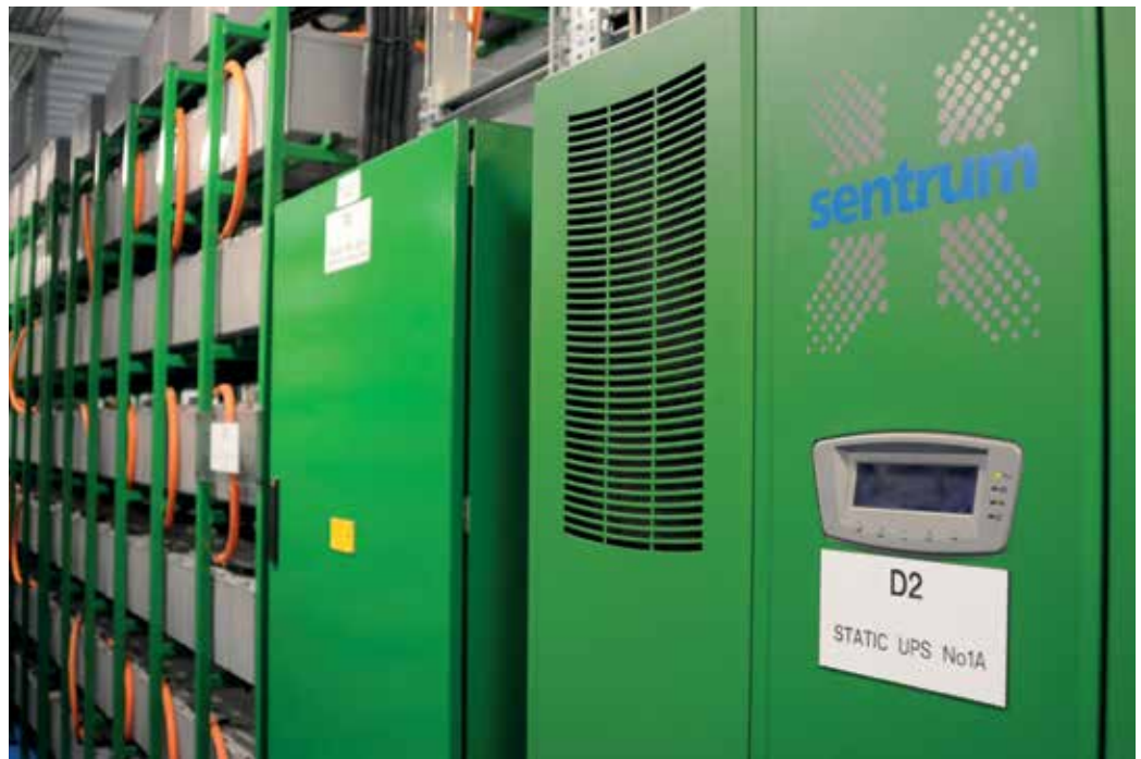
The UPS installation at Woking comprises 112 Eaton 9395 UPSs with ratings between 275 kVA and 825 kVA
